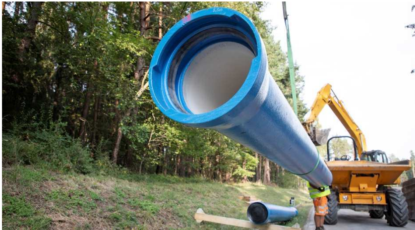
GJS Rohr DN 400 mm
